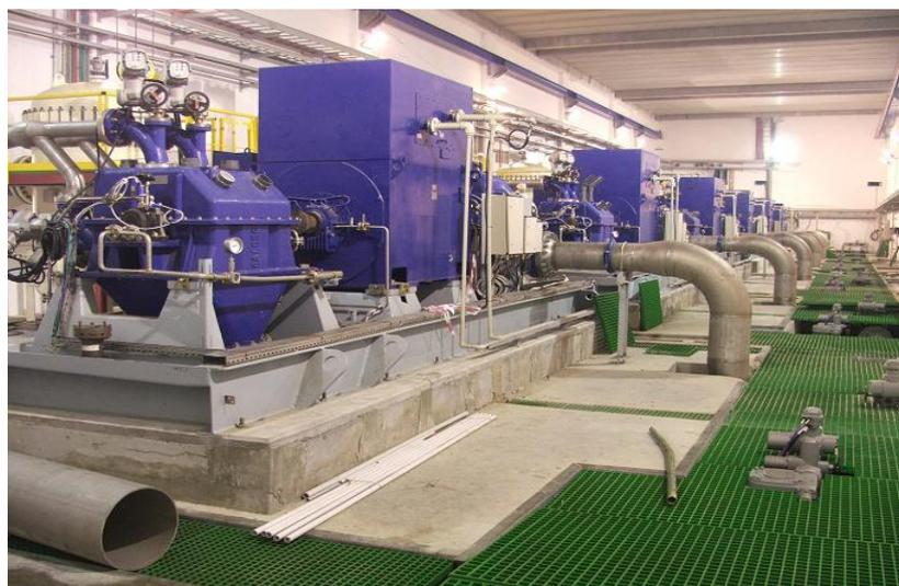
**Figure 2 A– Palmachim train include ERT+MOTOR+HPP**
