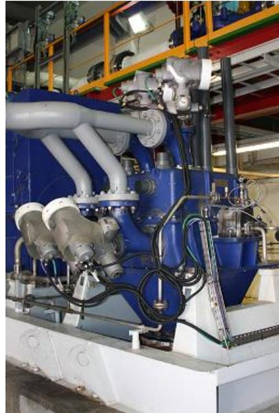
**Figure 2 – Palmachim Two-Runner ERT**
