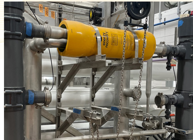
Photo courtesy of Kimley Horn and Associates, Inc.
