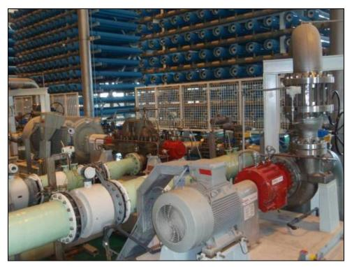
Figure 1 – High Pressure Pump, Circulation Pump and Membrane Array
