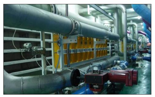
Figure 2 – PX Energy Recovery Device Array
