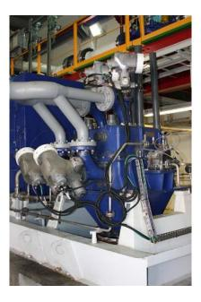
Figure 2 – Palmachim Two-Runner ERT
