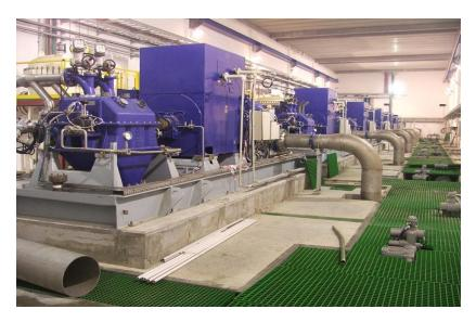
Figure 2 A– Palmachim train include ERT+MOTOR+HPP
