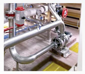
The turbocharger was integrated between the first and second stages to transfer the pressure energy from the second stage's reject stream to the second stage's feed stream. It acts as a booster pump between the stages, resulting in the same flux-balancing benefits, such as reduced membrane fouling.
