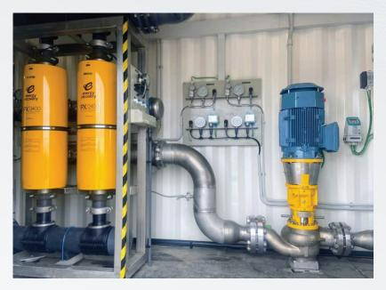
To achieve the aggressive performance targets of DESALRO 2.0, ITC turned to Energy Recovery, Inc. and its Q400 PX® Pressure Exchanger®, a proven solution for reducing energy consumption in desalination plants.
